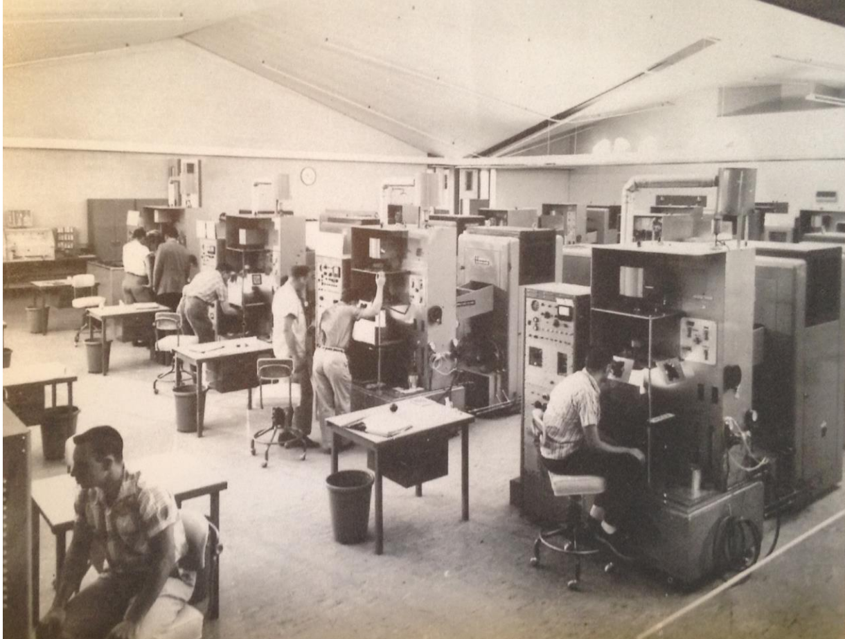
Figure 16. This image shows both the underside of the hyperbolic paraboloid roof and machinery that was used in the SC Building. The original caption reads: "Operators control the growth of silicon and germanium crystals, purer and larger than gems found in nature. TI operated the electronics industry's largest battery of the intricate machines in its new Semiconductor Components plant around 1958." Pirtle, 69.
