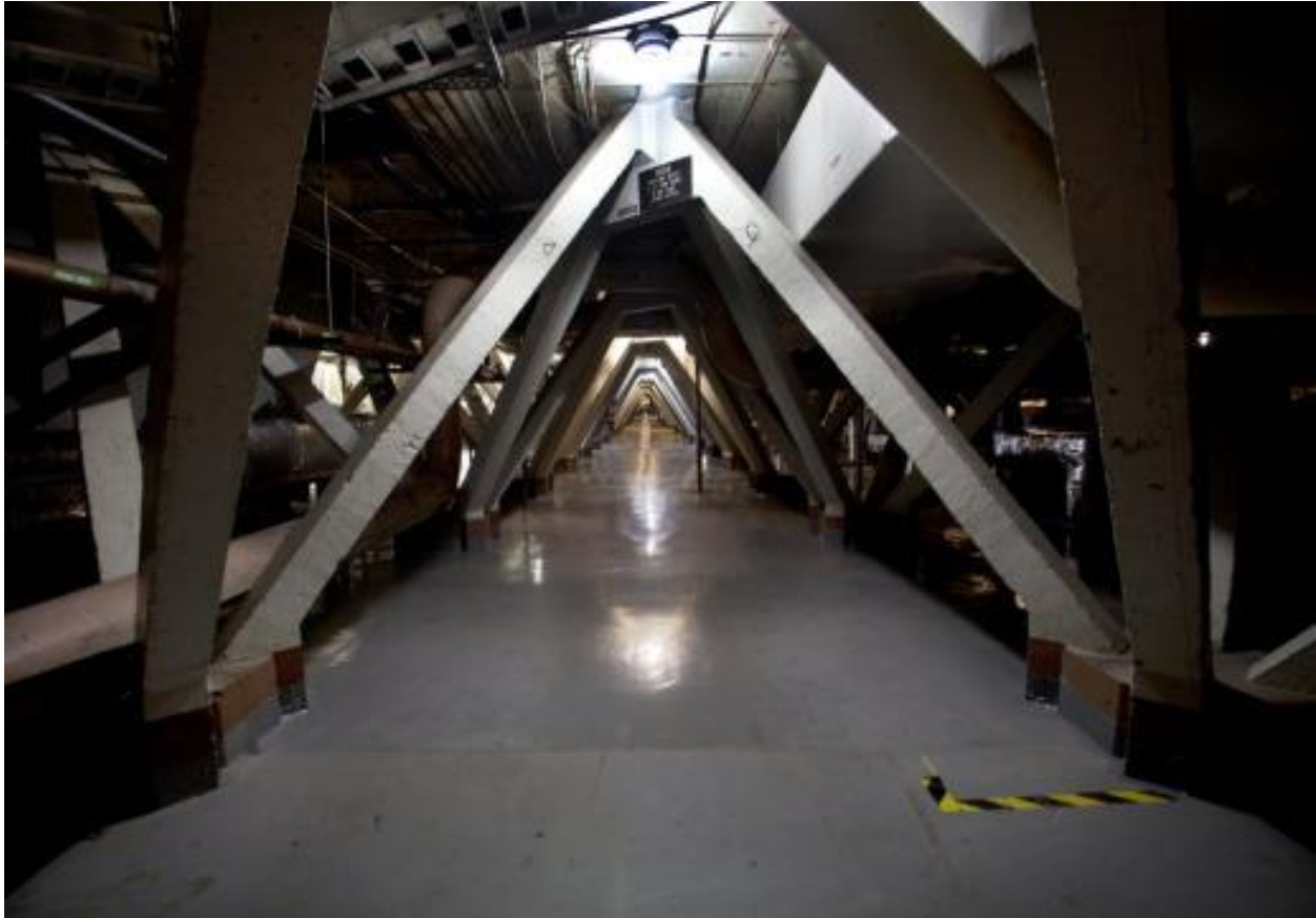
Figure 17. O'Neil Ford and Richard Colley, Texas Instruments Semiconductor Building, second floor. Photo by Nan Coulter, retrieved from Charissa Terranova, "O'Neil Ford's 1950s Texas Instruments building is still a haven for high-tech," FD Architecture Design , October 15, 2014. Accessed December 29, 2015. http://www.fdluxe.com/2014/10/infinity-beyond-inside-texas-instruments.html/#prettyPhoto .
